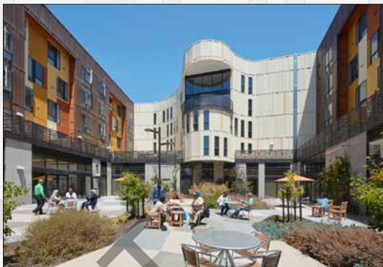
Dr. George W. Davis Senior Residence and Senior Center in San Francisco combines permanently affordable housing with a 1,300 m 2 neighbour-serving senior center, designed as a vibrant community hub rooted in local culture and certified LEED Platinum.
